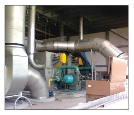
Exothermics was contacted by a major cheese manufacturer to provide an air heater that would deliver clean, heated process air for the operation of a new whey spray dryer. Exothermics' solution was a pair of Eclipse ER Indirect Air Heaters operating side-by-side. Not only do these air heaters produce clean hot air for this customer, free of combustion by-products and other contaminants, but they do so with impressive fuel efficiency.
